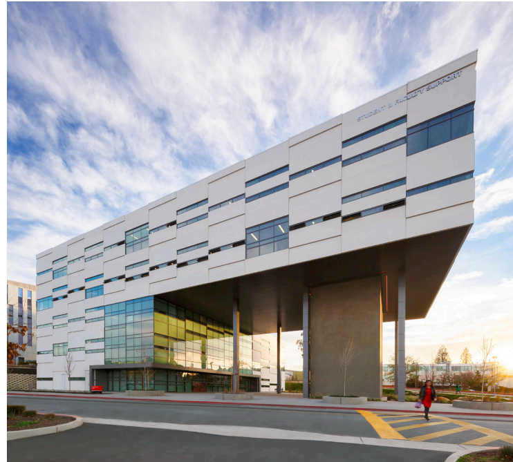
California State University–East Bay's Warren Hall features insulated C-CAPP (Clark Composite Architectural Precast Panel) panels, which were designed, fabricated, transported, and installed by Clark Pacific. One hundred thirteen of the panels run horizontally along the facade and provide sufficient insulation to help the building achieve LEED gold status. Photo courtesy of Costeaphoto.com.
