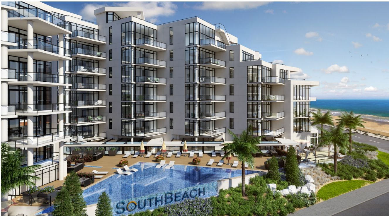
This new five-star, oceanfront, multifamily development in Long Branch, N.J., designed by James Monteforte of Monteforte Architectural Studio, uses Smith-Midland Corp. SlenderWall precast concrete building panels for their aesthetics, light weight, strength, durability, and energy efficiency. Courtesy of Costea Photography Inc.
